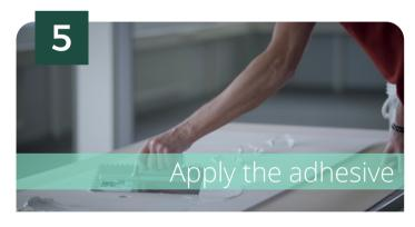
After cleaning the surface of the slab with a damp sponge, **apply the adhesive on the back of the panel** with the flat side of the trowel in straight lines using the **Back butter method**.
