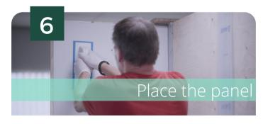
**Press the panel gently** onto the surface (use a pressing tool to help). When placing the panel, **ensure all the edges adhere to the surface**. If any adhesive seeps out, remove it immediately with a damp cloth.
