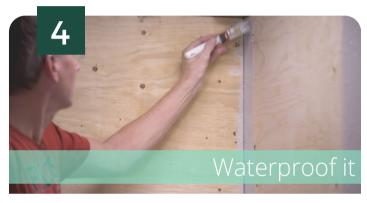
**Apply the 1st layer** (15 cm width) of the waterproof membrane in the vertical inner corner (the connection between wall and floor and the joint between the two slabs).
