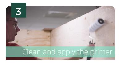
**Clean and levelled** the base walls and apply the recommended **Sustonable primer.**
