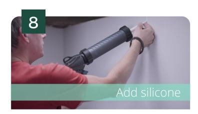
Add the silicon kit to the joints. Then, use a scraper to press the kit in the joint. Clean the panels where necessary. Let it dry and the work is done.
