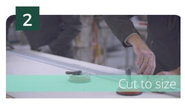
Use a **water-supplied cutting device** compatible with a diamond blade to cut the slabs. **Put the cutter guides on the panel**. Slowly, cut the panels into lengths.
