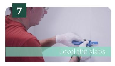
Level the slabs with a **levelling system** to prevent any movement of the panel during the adhesive's setting.
