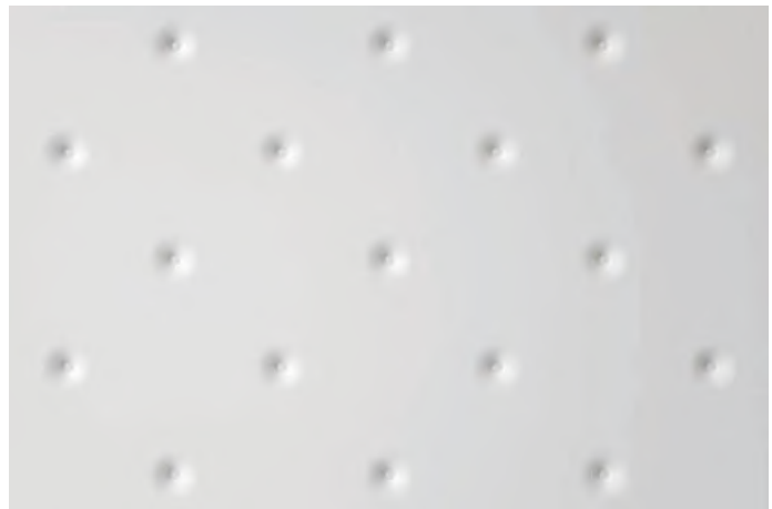
Wall Cladding Design of bubbles with air- and sound absorption holes Schönhauser Tor, Interior Wall Cladding; Berlin, Germany
