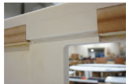
View of reinforcing block after finishing
