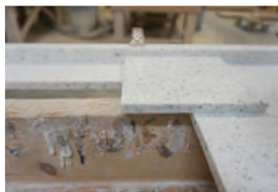
Close-up of reinforcing block in place
