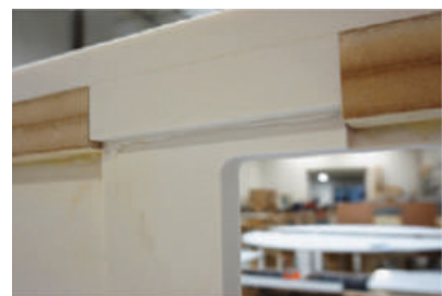
View of reinforcing block after finishing
