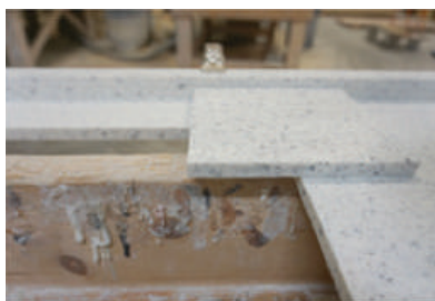
Close-up of reinforcing block in place
